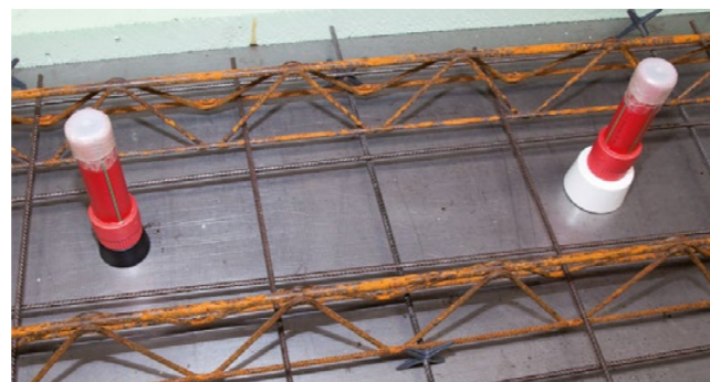
1. Type of connection: visible sprinkler
