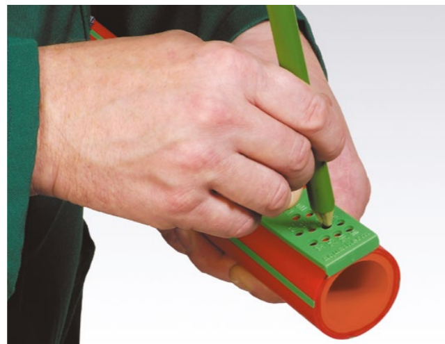
Marking of the welding depth
