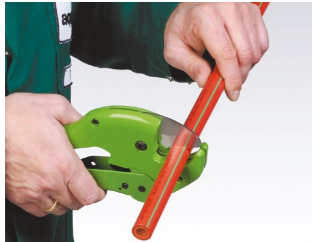
Cutting of the pipe
