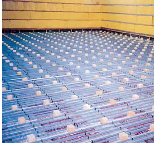
Tacker technique with pipe clamps
