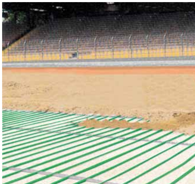
Placing of rails
