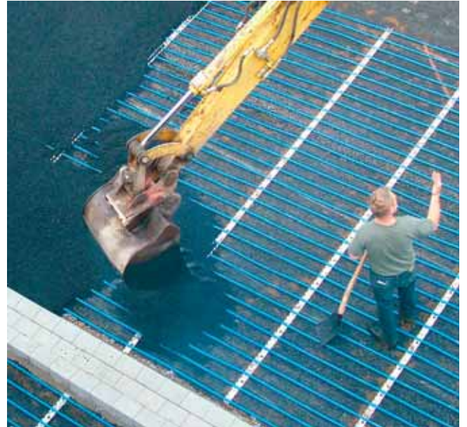
Open space heating system
