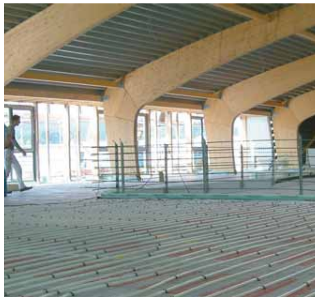
MAX-FITNESS-CENTER, Installing of sports floor heating system
