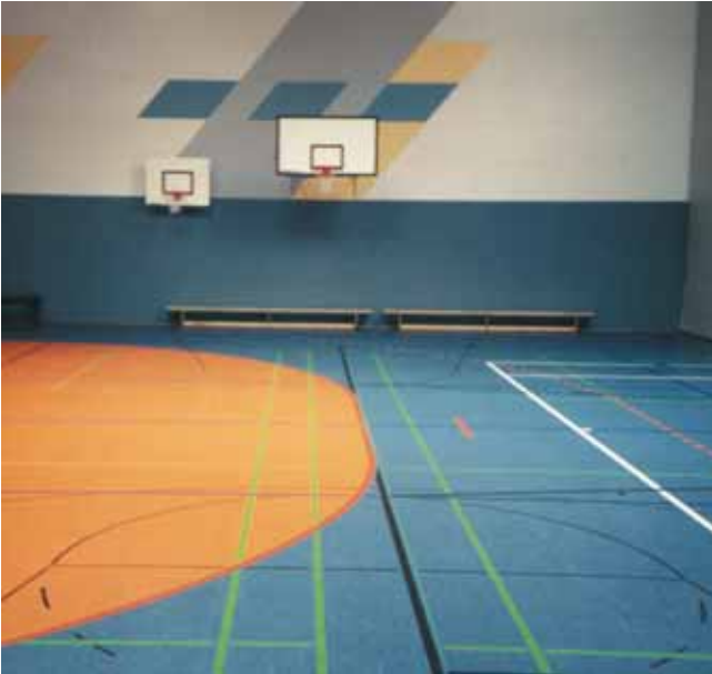
Finished sports hall with aquatherm® sports floor heating system with linoleum covering
