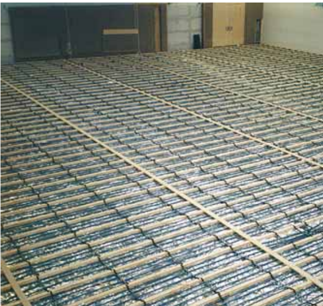
Laying with pipe suspension rail
