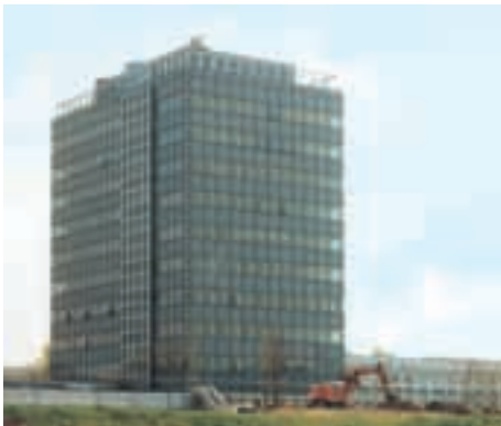
Pharmaceutical facility Hoechst AG (administration), Frankfurt am Main, Germany
