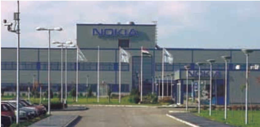
NOKIA production facility, Komárom, Hungary
