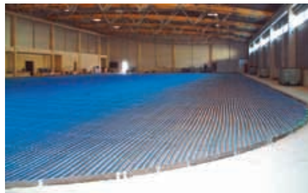
Ice rink Sonneberg (cooling surface laid with climatherm pipes), Germany
