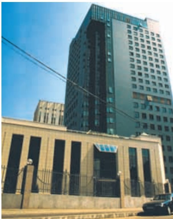
„Gazprom“ building, Moscow, Russia
