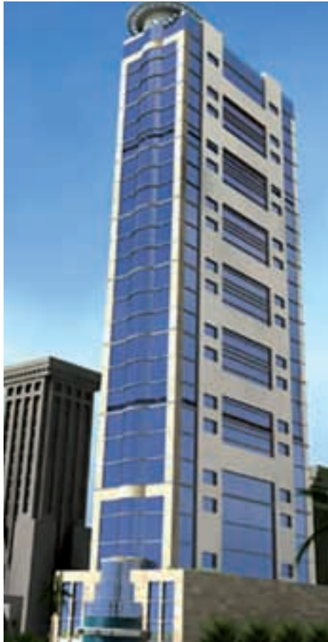
Flex Tower, Ras Al Khaimah, United Arab Emirates
