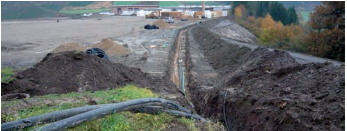
Saw mill, Josef Schmelter, Lennestadt-Oedingen, Germany
