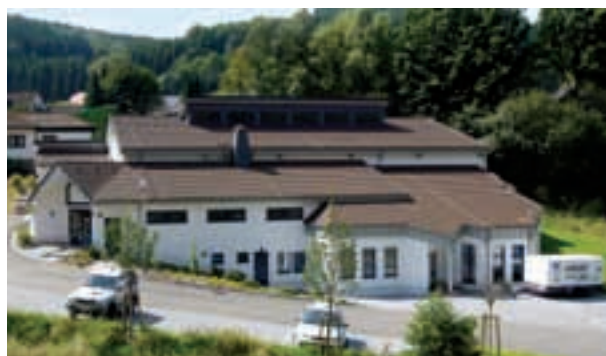
Sports hall Lichtringhausen, Attendorn, Germany
