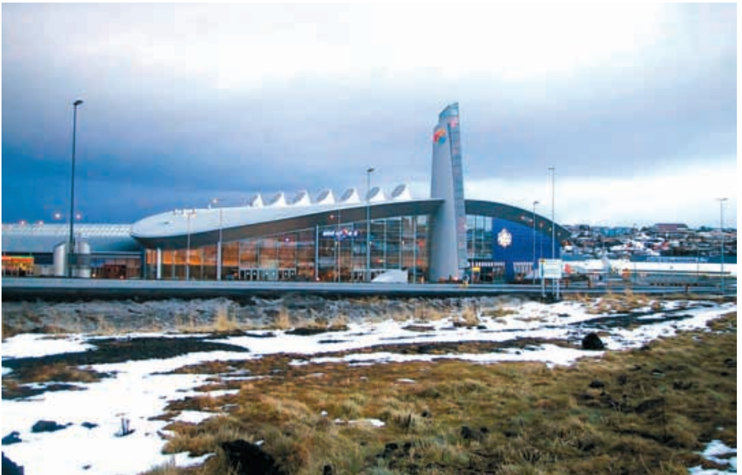
SMARALIND - Iceland's largest shopping centre (63.000 m 2 )
