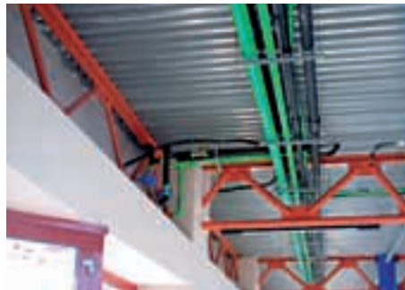
Millennium Stadium, Ceiling Installation
