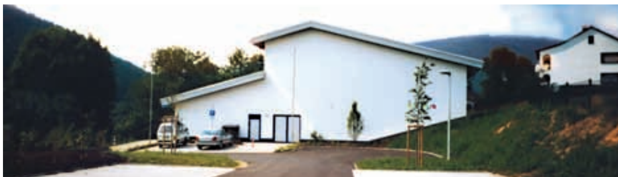
Sports hall Rönkhausen, Germany
