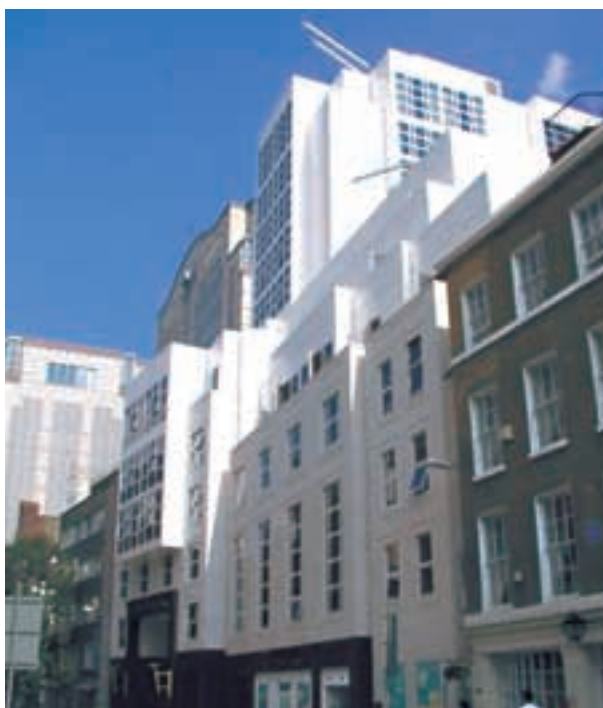
The Grange City Hotel is a spectacular new luxury 5 star hotel. The Grange City Hotel in London, England, is equipped with a sprinkler system made by aquatherm
