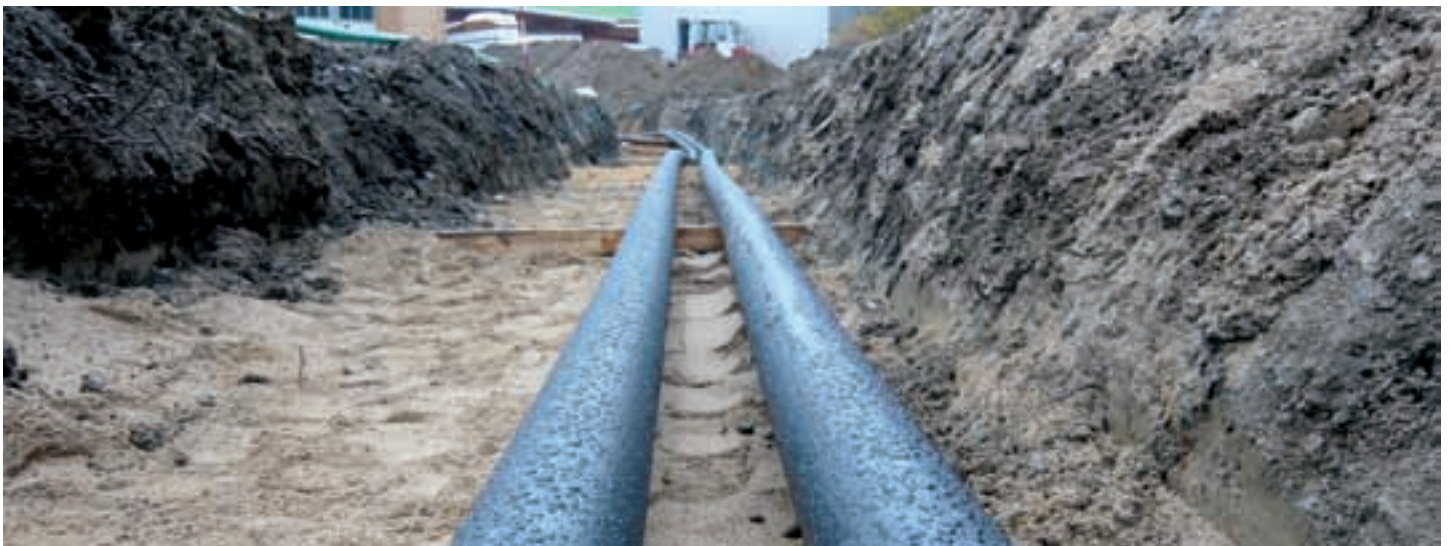
Underground service pipe with aquatherm ISO
