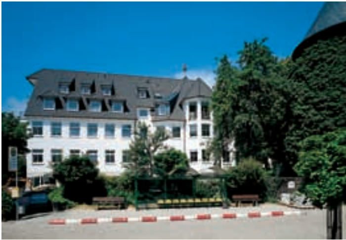
Residential and business building (AOK), Attendorn, Germany
