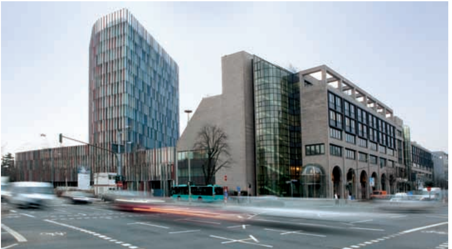
KFW Banc, Frankfurt, Germany (climasystem ceiling heating and cooling)
