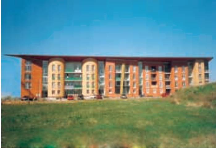
Residential building Parkstadt, Unterlindenbach, Germany
