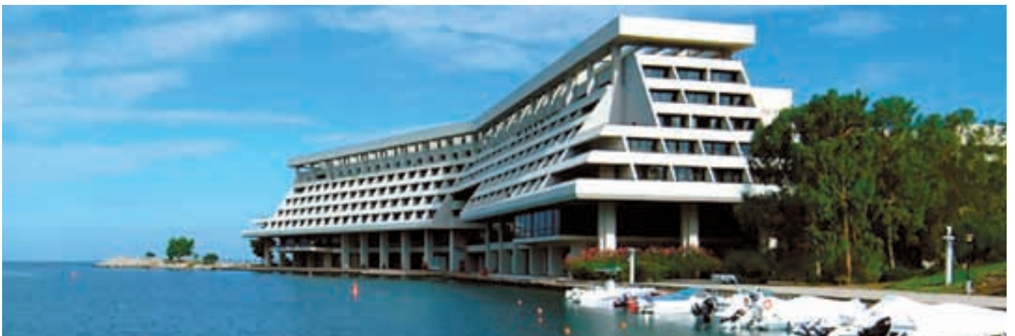
Hotel Melliton in Porto Carras, Greece. The top class hotel equipped with aquatherm pipe technology, has now secured itself a place in future European history books.
