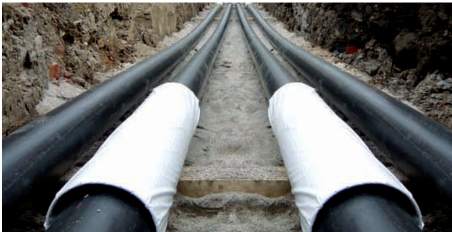
Underground service pipe with aquatherm ISO
