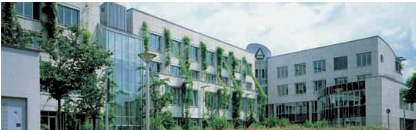
Agrippina insurance building, Kornwestheim, Germany
