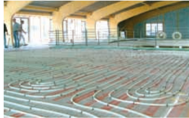
MAX FITNESS CENTRE, installing the sports floor heating, without...
