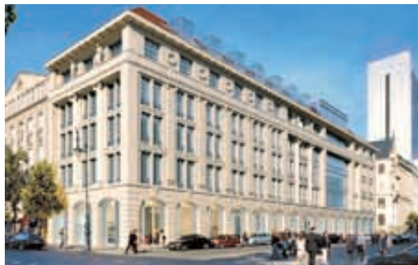
... and used as sprinkler system in the finished Römischer Hof ®
