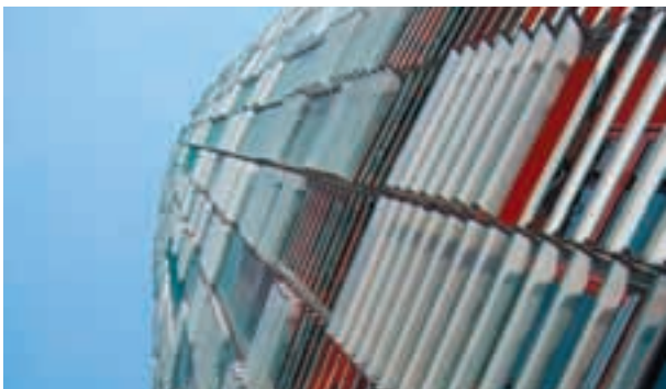
Thousands of narrow, louver glass panels enclose the reinforced steel façade of the Agbar Tower. They open outwards and provide shade.
