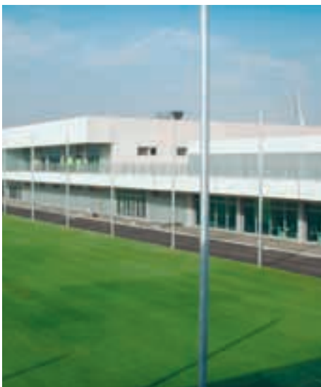
Team apartments, training centre and one of the soccer training fields as a model...
